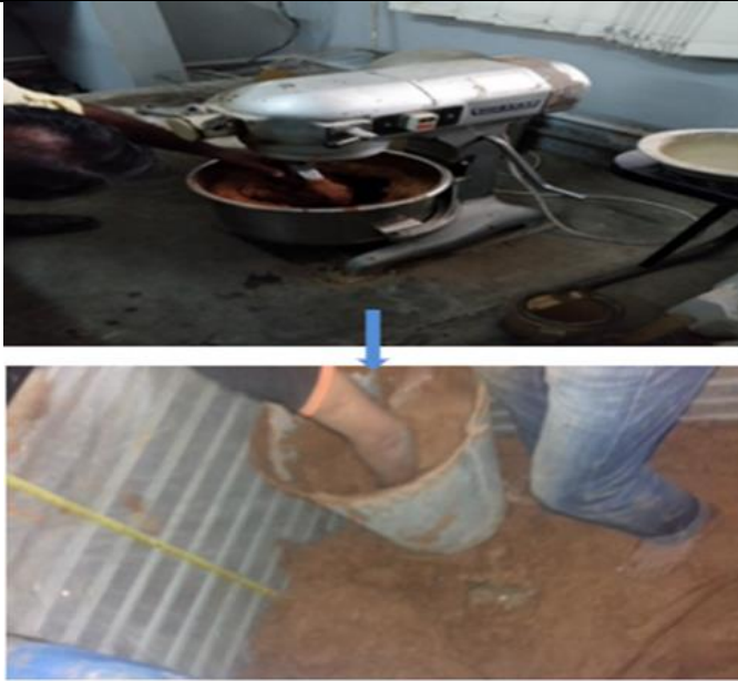
Figure 5. Preparation of clayey layer under embankment
